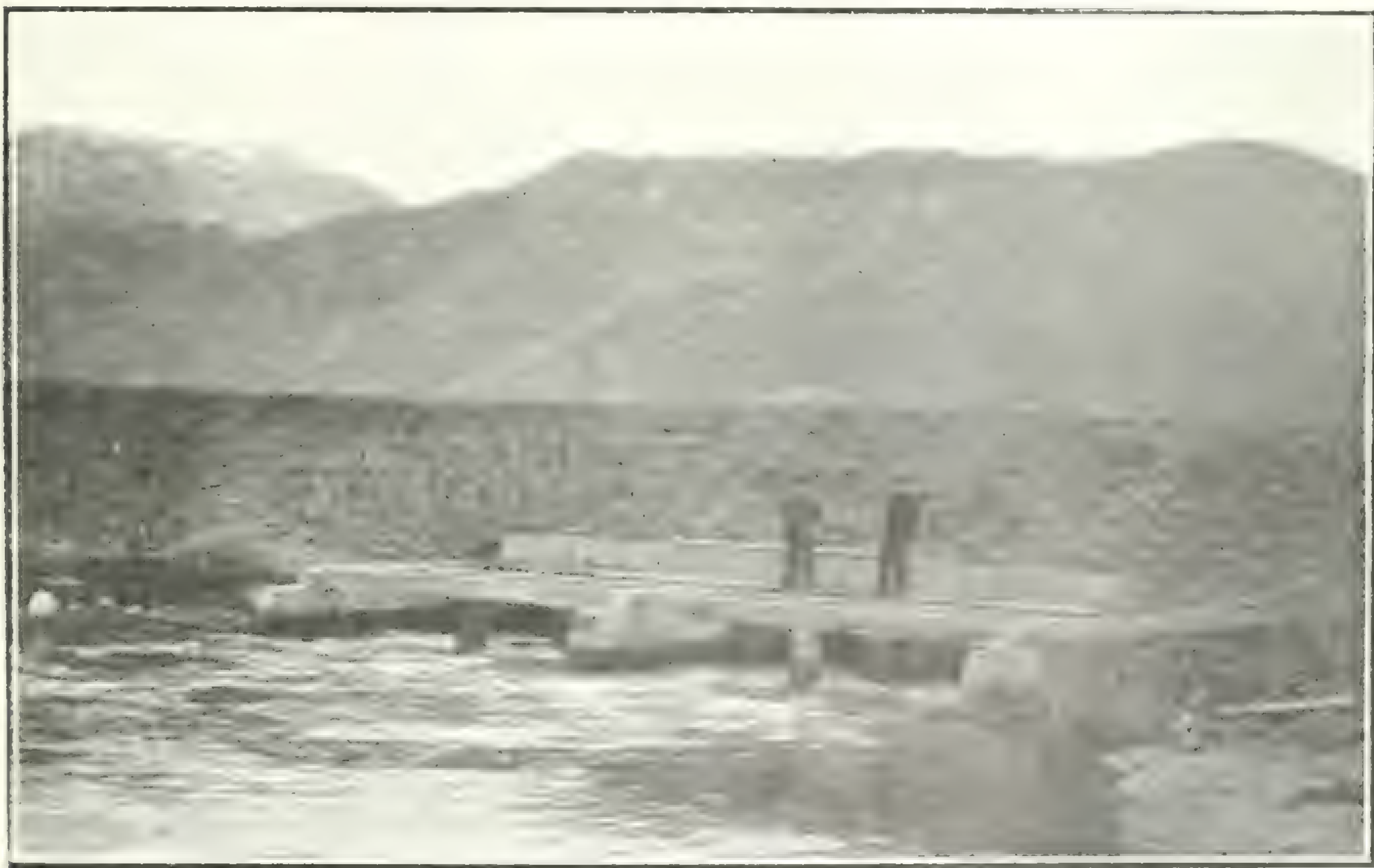
Reclamation—Pitt Meadows Dyke and Sluice Gates.
